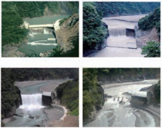
Figure 2. Sequence of photographs looking upstream at Barlin Dam and its failure in 2007. Note the exposure and extent of the reservoir sediment in 2005. The defense dam, which was critically damaged during Typhoon Aere in 2004, completely failed in 2006. (Photos courtesy of Taiwan Water Resources Agency, used with permission.)
